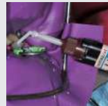
2. Core-Flo DC applied after use of Universal Primer™
